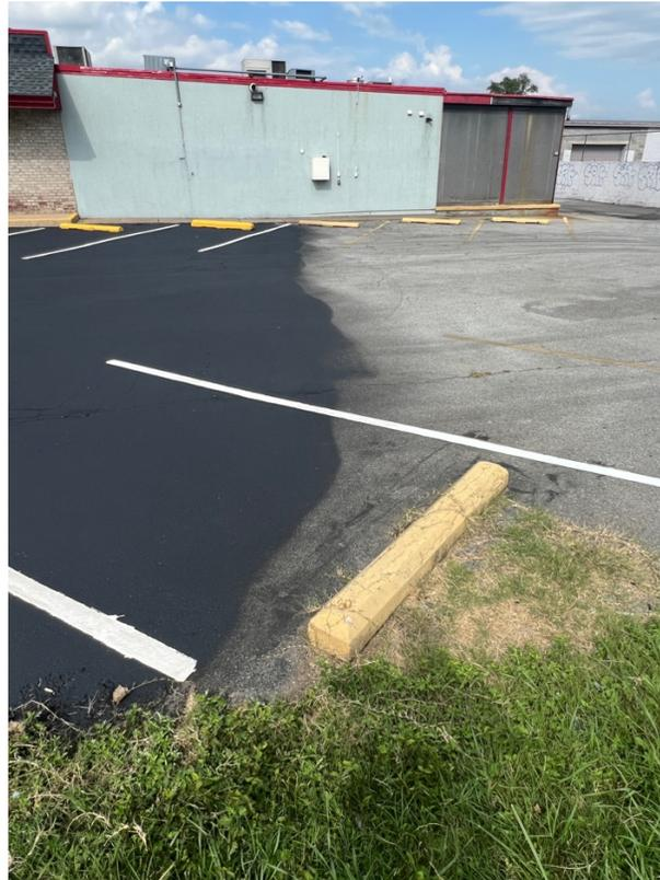
*The picture above is an example of a poor quality seal coating project a customer received from not properly qualifying a seal coating contractor.*
