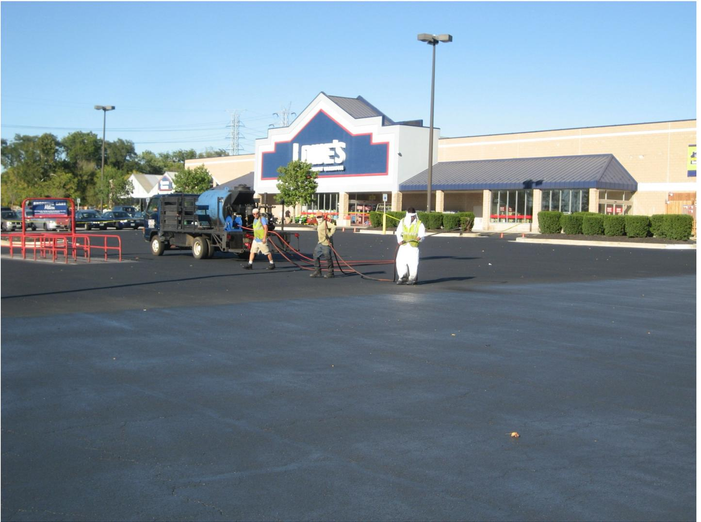
In this verification picture it is visibly evident of the 2<sup>nd</sup> coat of pavement sealer being applied.
