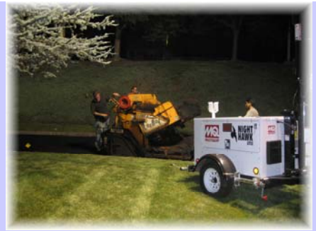
Asphalt Paving Being Performed Under A Light Tower For Quality Control
